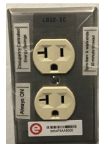
Switched receptacle with labels
