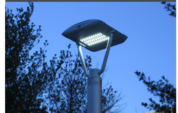
LED exterior fixtures often have opaque tops and produce no uplight. This fixture has a U0 uplight value. Photo credit Michael Myer, PNNL
