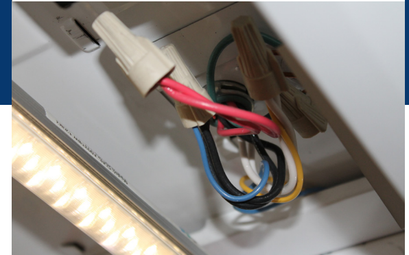
Type B TLEDs are directly wired to line voltage. Photo credit Michael Myer, PNNL
