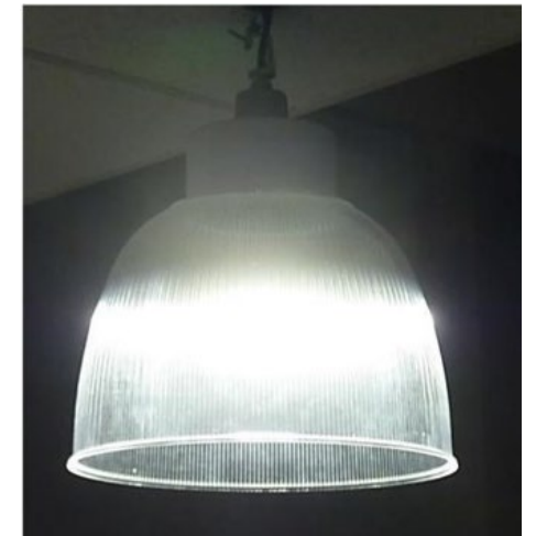
Retrofit kit has a solid backing and no longer illuminates the ceiling.
